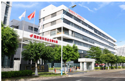
"WePure" Headquarter located in Guangdong
